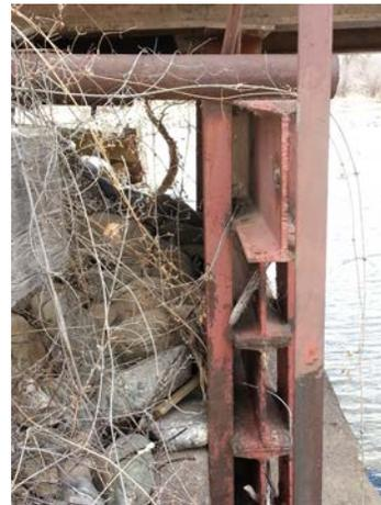
The east bridge abutment has experienced deterioration and settlements. Since the abutment is retaining soil, the lateral loads applied to the abutment has caused the top to deflect towards the river. Although the east abutment has been performing over the years, the abutment capacity is suspect and does not meet current AASHTO codes.
