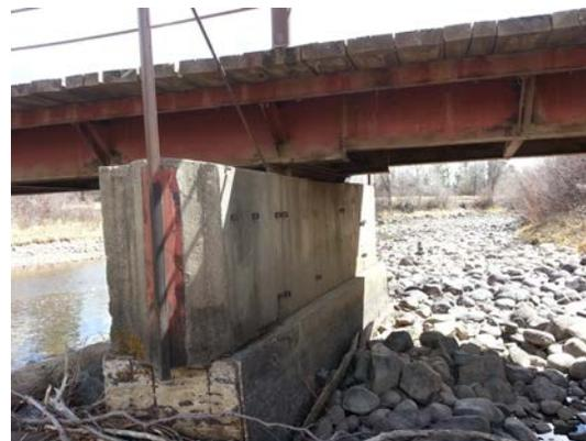
Cantilevered Bridge Deck Ends
