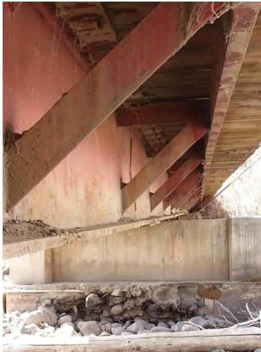
Bridge Steel Bracket Support at Deck Cantilever
